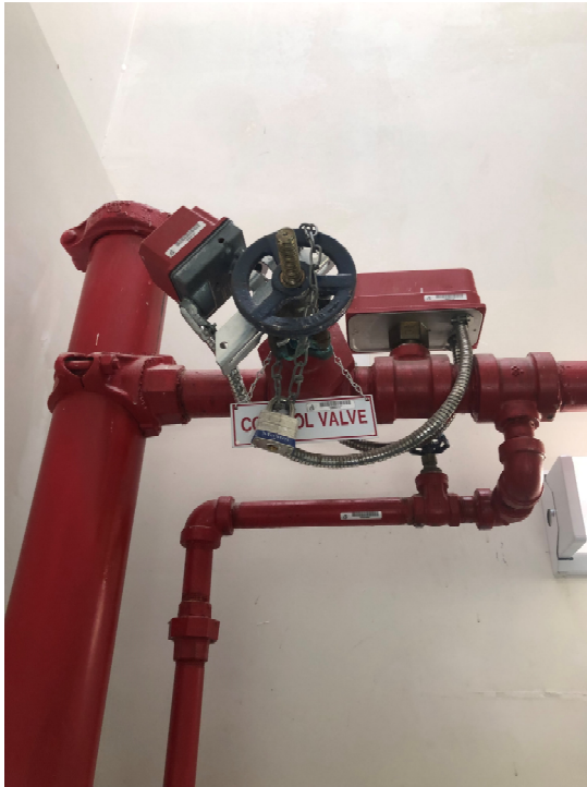
Floor Control Valve Assembly
